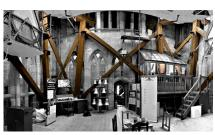
The large wooden beams are made of pitch pine and form an internal tower 56 feet (18 metres) tall. It rests on the base of the tower's stone piers and is keyed into the tower walls. This massive wooden structure is known
