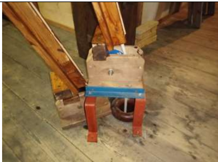
29 Sep 2020 – Bell test rung from carillon room. Rope chutes installed, with pulley-over-pulley arrangement. New sliderway made and bolted to framework. New stay created from a spare one.
