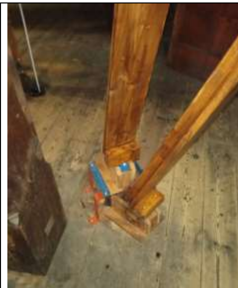
29 Sep 2020 – Bell test rung from carillon room. Rope chutes installed, with pulley-over-pulley arrangement. New sliderway made and bolted to framework. New stay created from a spare one.
