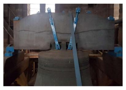
This picture shows the cathedral's bourdon bell which hangs with the sixteen ringing bells 160 feet (49 metres) up in the tower. This headstock supports the bourdon which weighs over 80 hundredweight (4072 kg). However, our bourdon bell does not swing. The bell is struck by a large hammer to sound the hour every day between 07:00 and 22:00. It can be chimed on mournful occasions.
