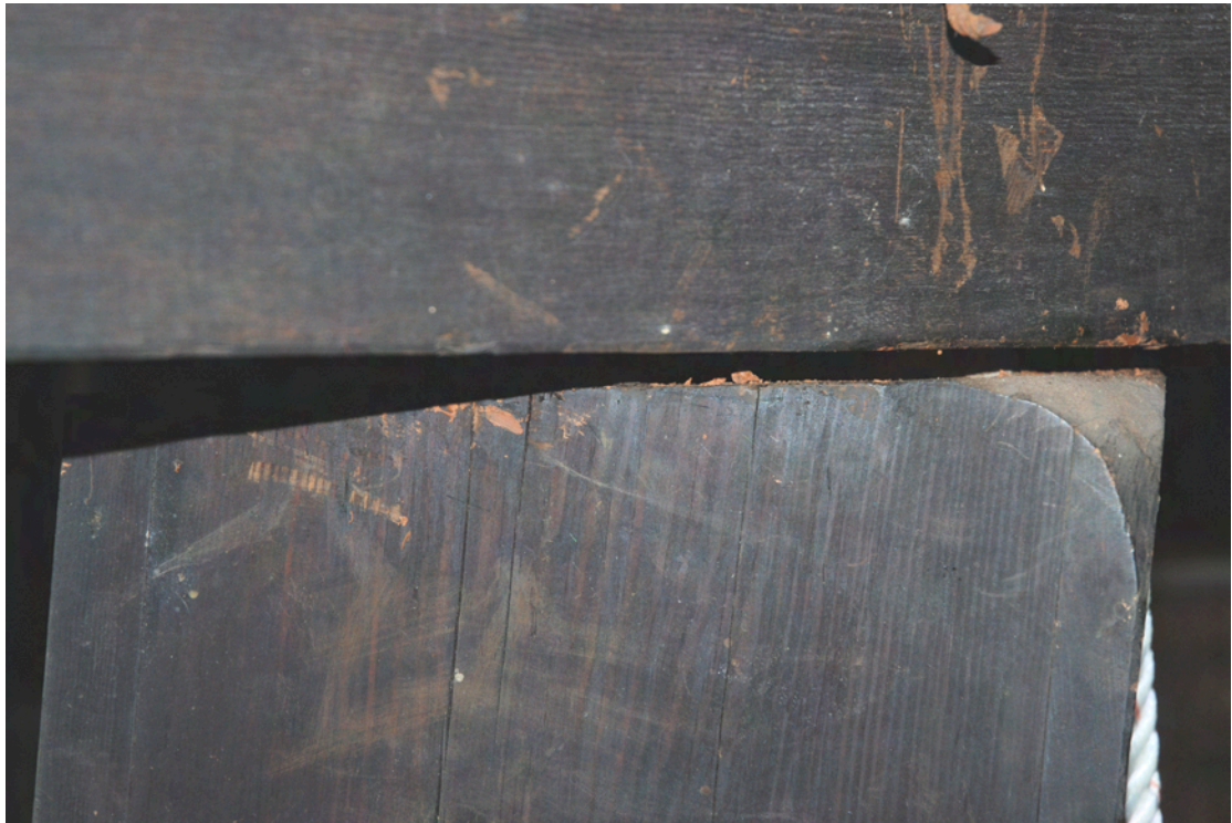
Tapered joint at top of Wigwam post
