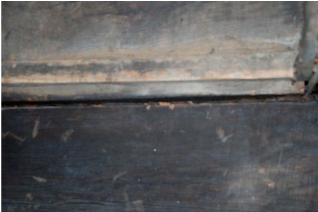
Complete lack of contact between bell frame and foundation beam
