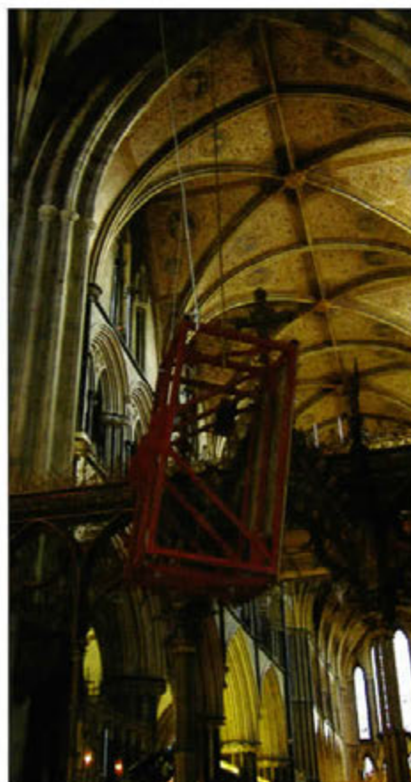
Frame going up to the tower trapdoor
